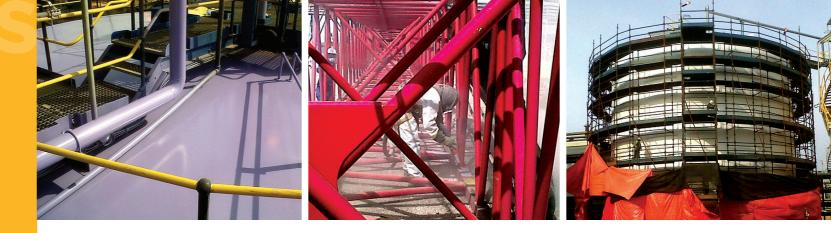
The company has a range of Acid Proofing and Corrosion Protection Lining systems from Epoxy Novolac FRP Lining systems, resin screeds up to 9mm thickness and Acid Tiles and Bricks from 15, 25, 38, 51, 65 & 76mm thick. Ensuring the concrete and steel tanks are protected against corrosion to extend the life expectancy of the structure. Suitable for Precious Metal Refineries, Fertilizer plants, Acid plants, Paper Mills, Chemical Processing Plants and any area exposed to chemicals.
