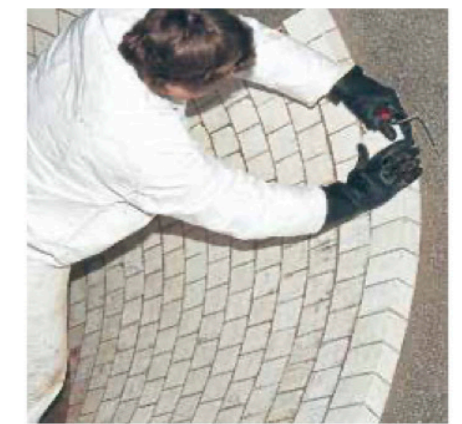
Kalenborn service solves wear problems on site
