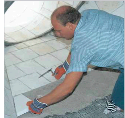
KALCOR lining of a hopper in the sinter dust collector of a steel mill
