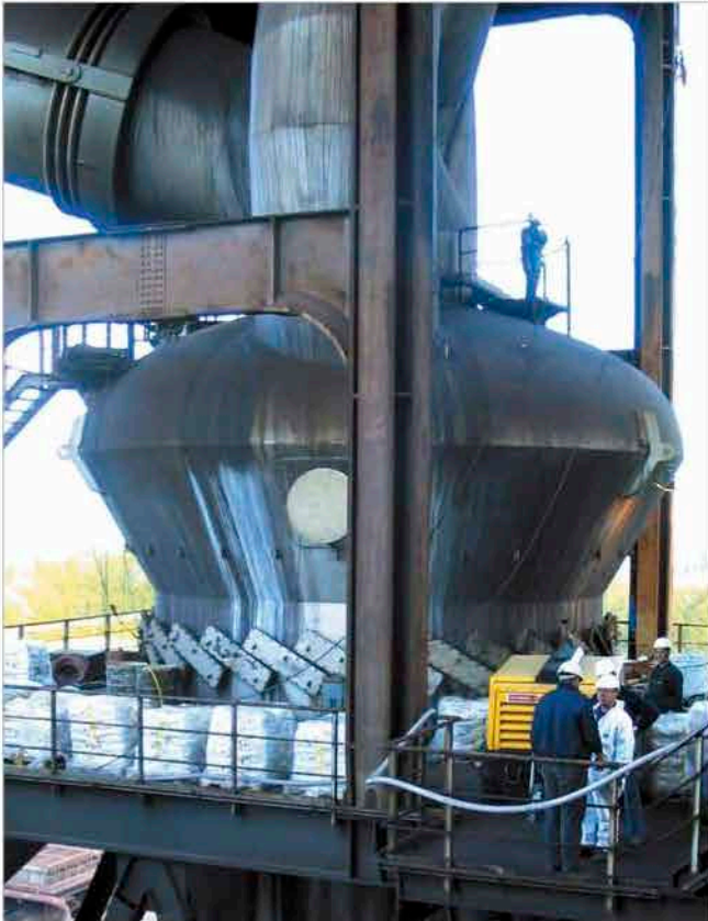
Scrubber inlet in a steel plant lined with sprayed-on KALCRET-BTS hard compound
