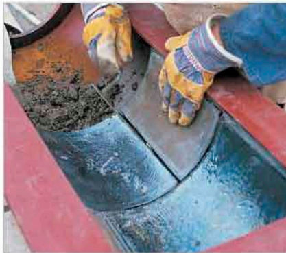
Setting in cement mortar
