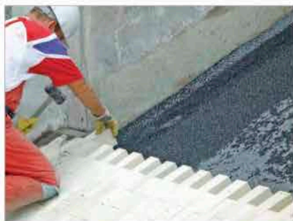
High temperature KALCERAM-K chute in a coking plant provides good sliding properties even at high temperatures
