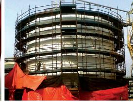
The company has a range of Acid Proofing and Corrosion Protection Lining systems from Epoxy Novolac FRP Lining systems, resin screeds up to 9mm thickness and Acid Tiles and Bricks from 15, 25, 38, 51, 65 & 76mm thick. Ensuring the concrete and steel tanks are protected against corrosion to extend the life expectancy of the structure. Suitable for Precious Metal Refineries, Fertilizer plants, Acid plants, Paper Mills, Chemical Processing Plants and any area exposed to chemicals.
