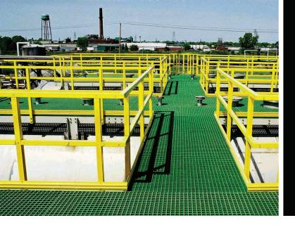
Fibreglass Reinforced Plastic (FRP) is a composite material made of a polymer matrix reinforced with fibres, usually glass fibres.
