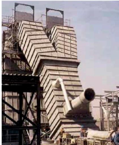
Cooler waste gas pipe lined with KALCRET BNY hard compound
