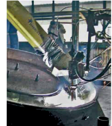
Kalenborn Service solves wear problems on site
