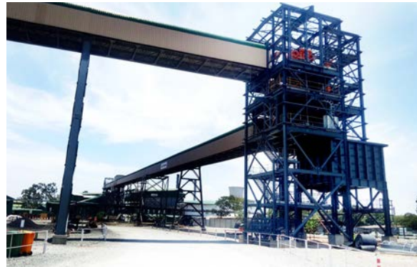
STRUCTURAL, MECHANICAL, PIPING, & PLATEWORK (SMPP)
