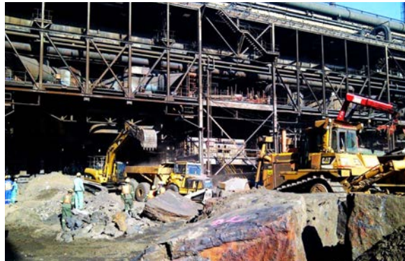
FURNACE DEMOLITION SERVICES
