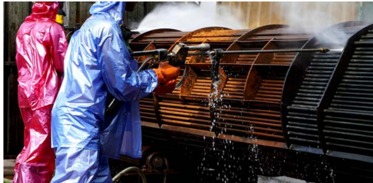
HP & UHP WATER BLASTING
